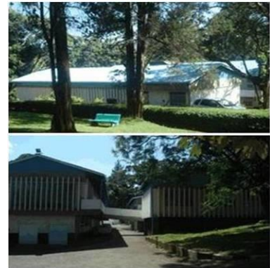
Part of CEBIB office and Labs
